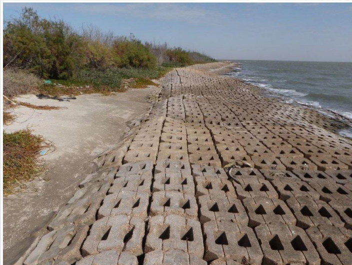
Figure 13. Articulated concrete mat revetment along northeast shoreline of Sundown Island
