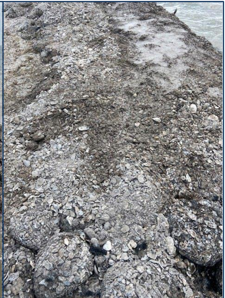
Photos 9 & 10: Project Area with Stacked Shell-Filled Mesh Bags Topped with Shell Hash
