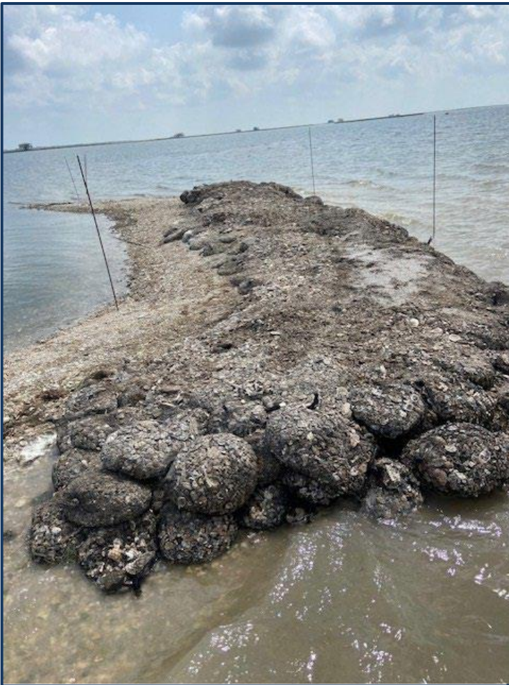
Photos 9 & 10: Project Area with Stacked Shell-Filled Mesh Bags Topped with Shell Hash
